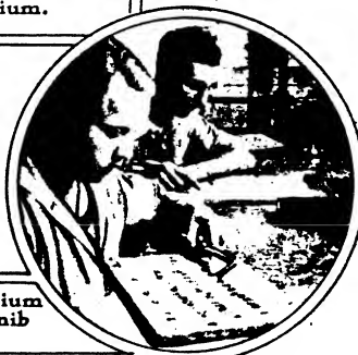
The 14K gold nib is tipped by hand with the hardest native iridium.
